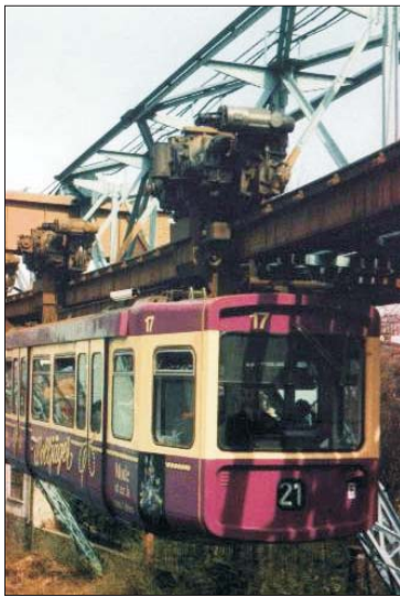
Fig. 1 • Suspension railway in Wuppertal
