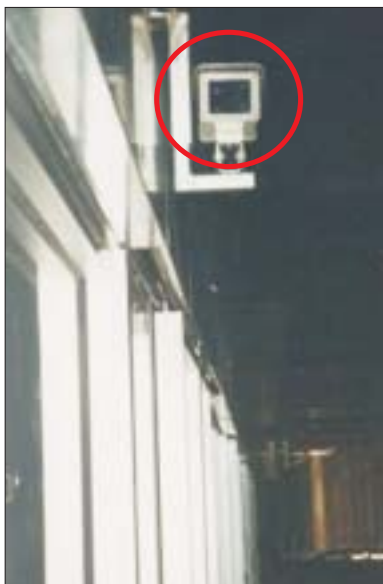
Fig. 4 • Kuala Lumpur Aiport terminal - ERL door control signals are transmitted from the train to the platform
