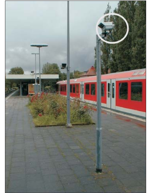
Infrared - Presence Detector FLG 10-20
